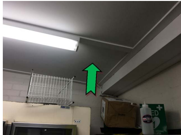
Photo 2. Interior, throughout, ceiling – non asbestos-containing fibre cement sheeting.
