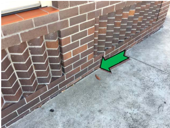
Photo 1. Exterior, throughout, ground, expansion joint – non asbestos-containing construction mastic.
