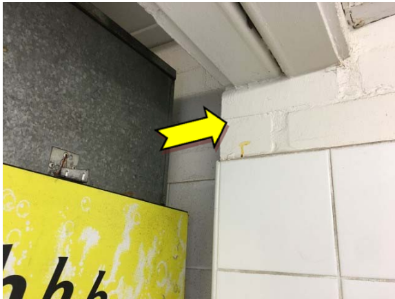
Photo 3. Interior, throughout, walls – suspected lead-containing cream upper paint system.
